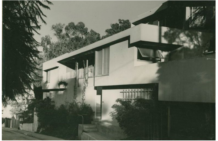
The Falk Apartments seen from Lucile Ave. circa 1943 (photo by Julius Shulman, courtesy of the R. M. Schindler papers, University of California, Santa Barbara )
