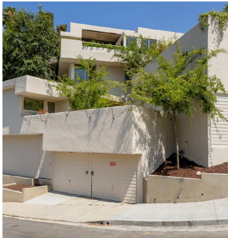
The Falk Apartments seen from Lucile Ave (photo by Cameron Carothers, courtesy of Dwell )
