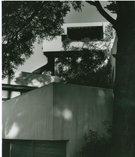
The Falk Apartments seen from Carnation Ave. circa 1943 (photo by Julius Shulman, courtesy of the R. M. Schindler papers, University of California, Santa Barbara )
