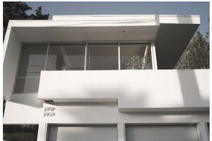
Guest house façade detail (photo by Larry Schaffer )
