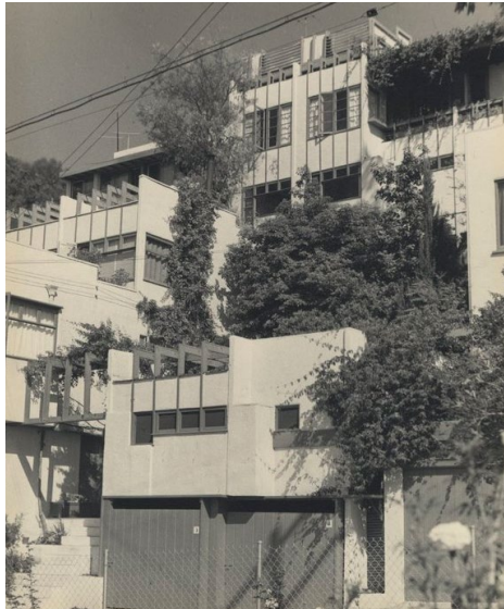
Façade (photo by Julius Shulman, courtesy of the Art, Design & Architecture Museum, University of California, Santa Barbara )
