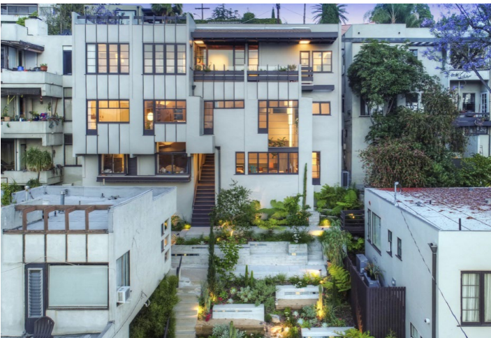
Back façade (photo by Charmaine David, courtesy of Manola Court )
