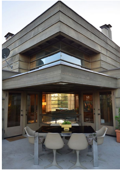
Back terrace (photo by Leelah Foster, courtesy of HGTV )
