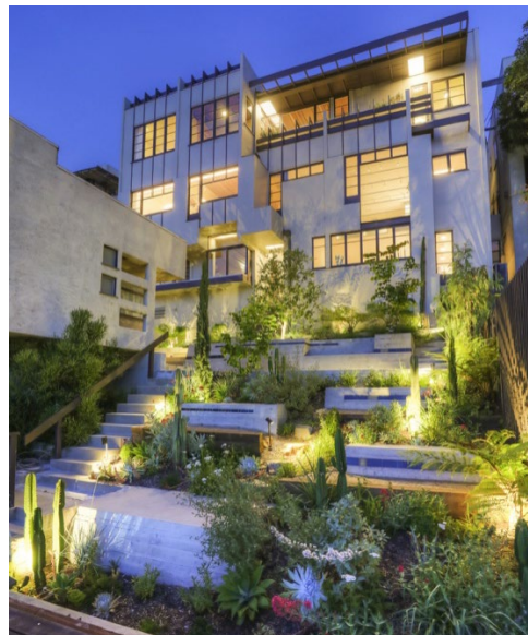
Overview of the penthouse, music room, maid's room and central courtyard (courtesy of Manola Court )
