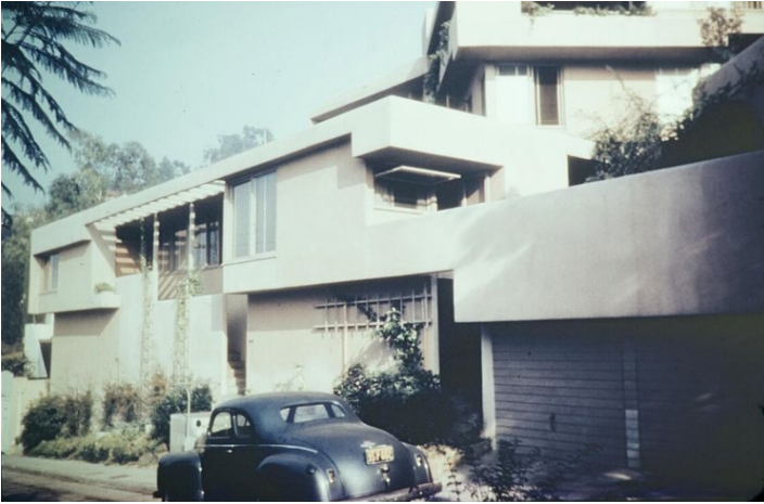
Falk Apartments (photo by Dr. Fritz Block, courtesy of USC Libraries)
